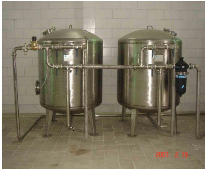
Stainless steel filters tanks of sand and active charcoal and also polycarbonate disc filter with related piping system
