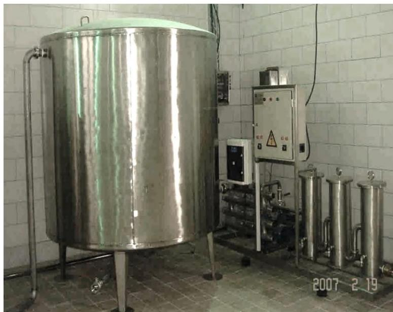
Stainless steel pre-treatment tank and UV pipe rows, buster pump and Micro filter cylinders
